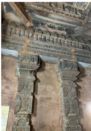
Photo 21: Column and beam
