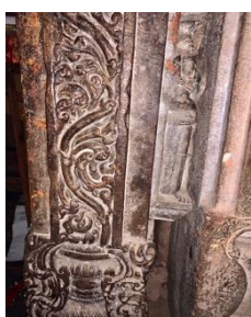
Photo 18: Left jamb of door no. 2
