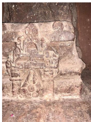
Photo 36: Base of pillar
