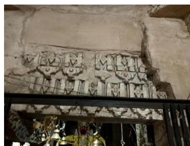
Photo 20: Lintel over door no.2
